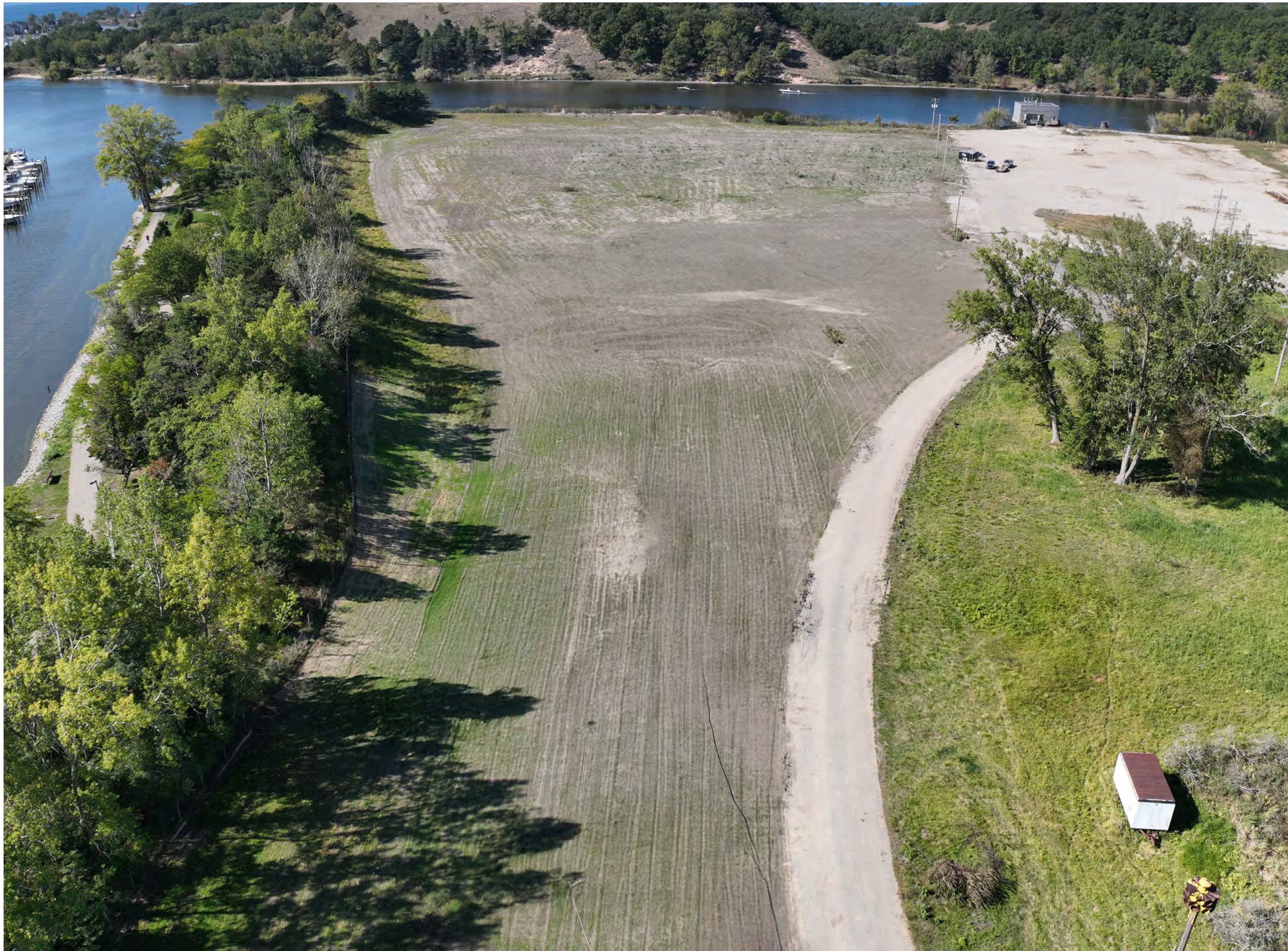
Full site view of the coal pile project area, looking west.
