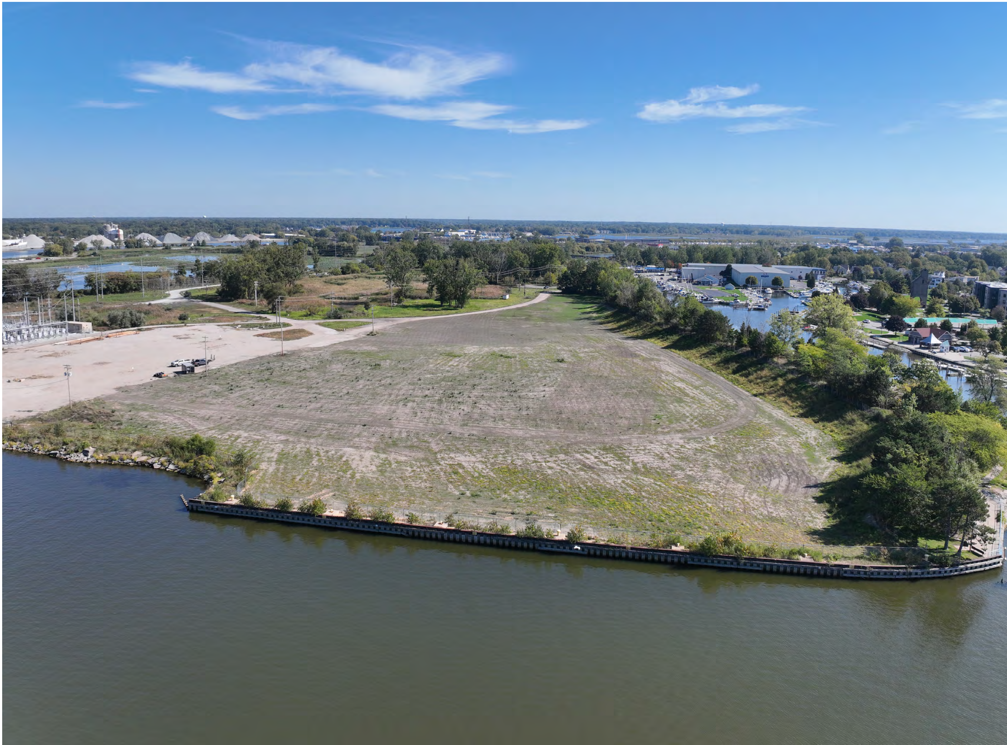
Full site view of coal pile project area, looking east.
